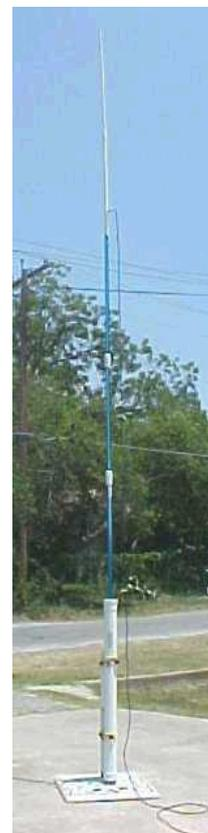
Take the 1092mm long x 75mm pvc sewer pipe and clean off both ends. Coat one end of the pipe with the all purpose cpvc/pvc cement and quickly install the 75mm end cap by pressing it on to the end. You must do this quickly as the solvent (cement) dries very quickly. Apply the same cement to the other end of the pipe and install the threaded sewer cap adaptor in the same manner.
